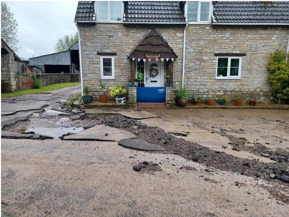
Figure 22 Image showing property in Queen Camel following flooding on 9th May 2023
